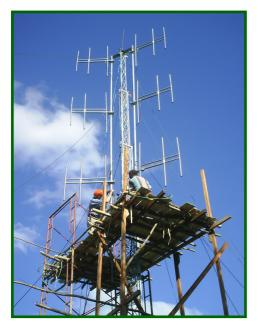
Step by step, the eight elements and the antenna cable (through splitters attached with tie-raps) were attached to the new construction. After every two elements, the tower was raised to the next level. The antenna elements were attached in an angle and direction that allows the signal to reach as many villages within Viguegue District as possible (away from the sea). The tower was growing higher bit by bit, and became visible for the people down at the market.
