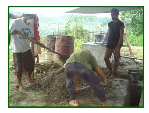
Immedeately after the welded foundation was delivered, the Concrete Team started mixing the concrete and filled up the hole. Two men kept the concrete moving by stirring it with long sticks. This is to release air and upgrade the concrete's quality. As they reached the instructed level, Bas monitored placing the iron foundation. Then the workers added concrete and worked until way after dark, as all concrete had to dry in one massive block. It takes at least two days to dry.
