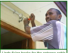
Lindo fixing hooks for the antenna cable
